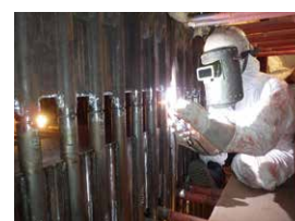
Replacing boiler tubes
