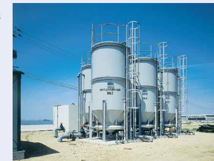
Upflow moving-bed sand filtration system
